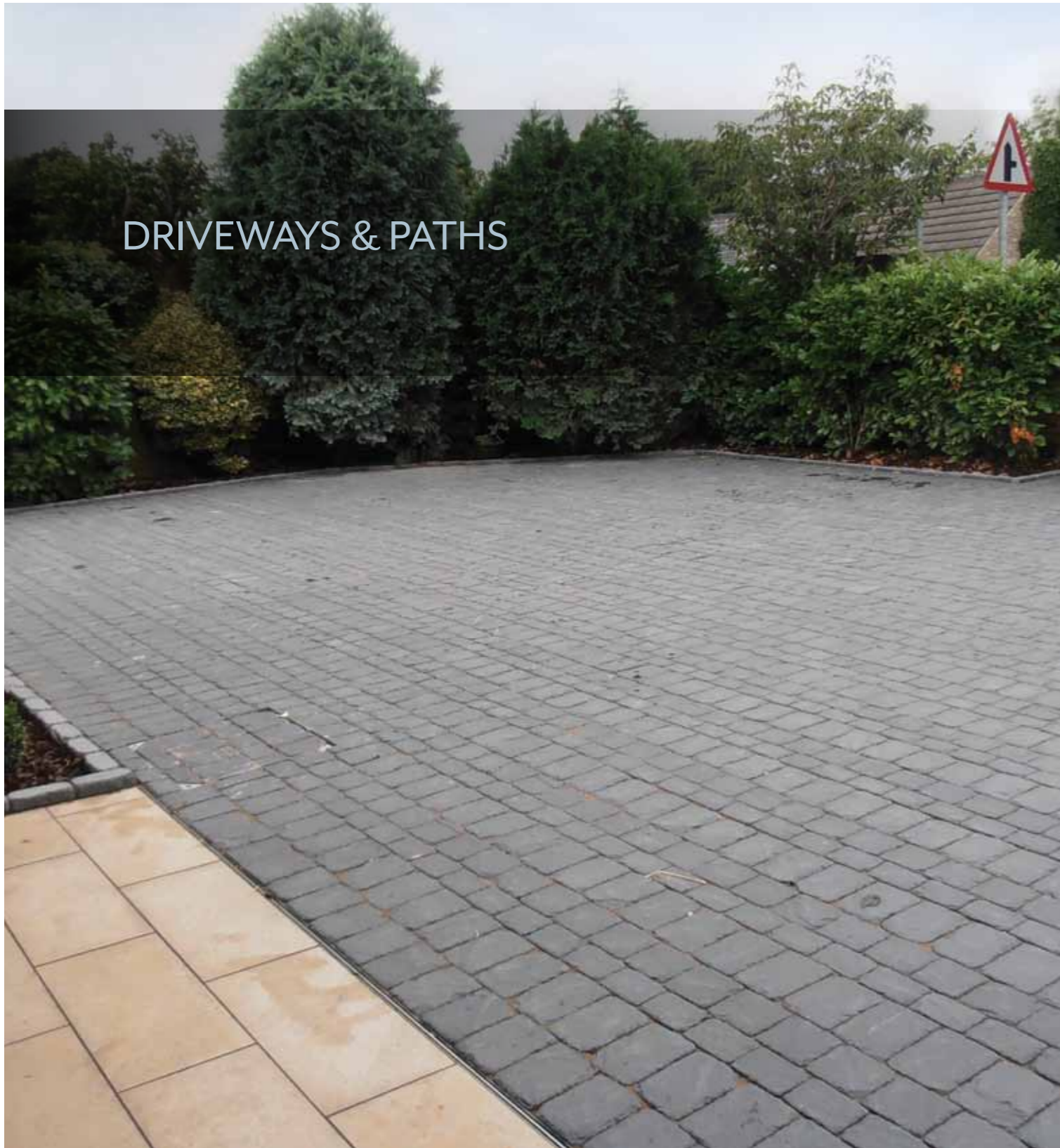
Residential Project using 3 sizes of the British Kirkby Blue Tumbled Stone Setts, laid on a flexible jointed screeded bed.
